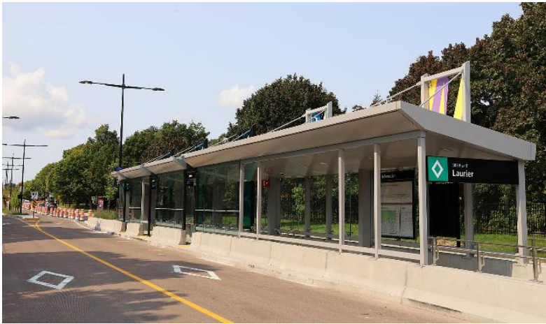
Bus rapid transit corridor in Montreal (Canada)
